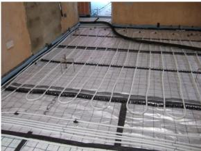
Under floor heating pipes were laid in a self adhesive rail system directly on to the multi foil insulation and Gridboard, the pipes were filled with water and pressure tested.
