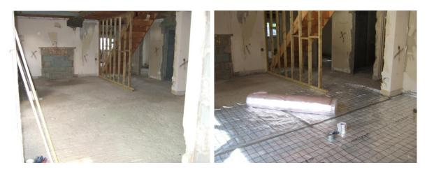
This is the floor after the removal of the old screed and with the new multi foil insulation being laid. The joints in the insulation were first taped together with an insulating foil tape and then the polythene layer was also sealed, a 10mm thick foam expansion strip was installed around the perimeter and internal walls, this is to allow for any thermal movement within the building or the screed.
