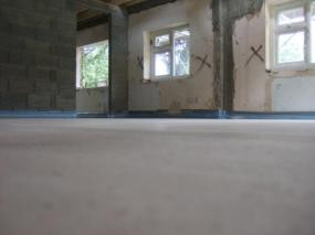
The screed was then poured at a depth of around 50mm bringing the finished floor level back up to roughly the same height as the previous floor.
