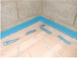
All edge details and penetrations in the concrete slab must be fully sealed to prevent screed leakage prior to handing over the floor for screeding.
