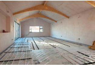
Under floor heating pipes must be filled with water and pressure tested before screeding commences.
